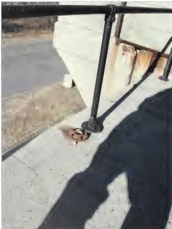
Figure 5.12. View looking west at safety railings, Battery Granger. The existing railing system at Battery Granger displays successive generations of railing components and repairs (Olmsted Center, January 2009).
